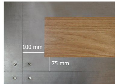
Figure 2: Location of 1000 x 150mm tile, which must be offset by 75 mm and 100 mm from edges of a raised access panel
